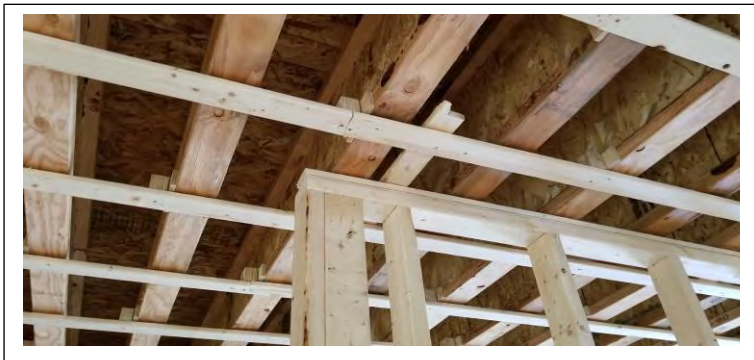
Wood furring decoupled on HushFrame Raft connectors. Simple.
