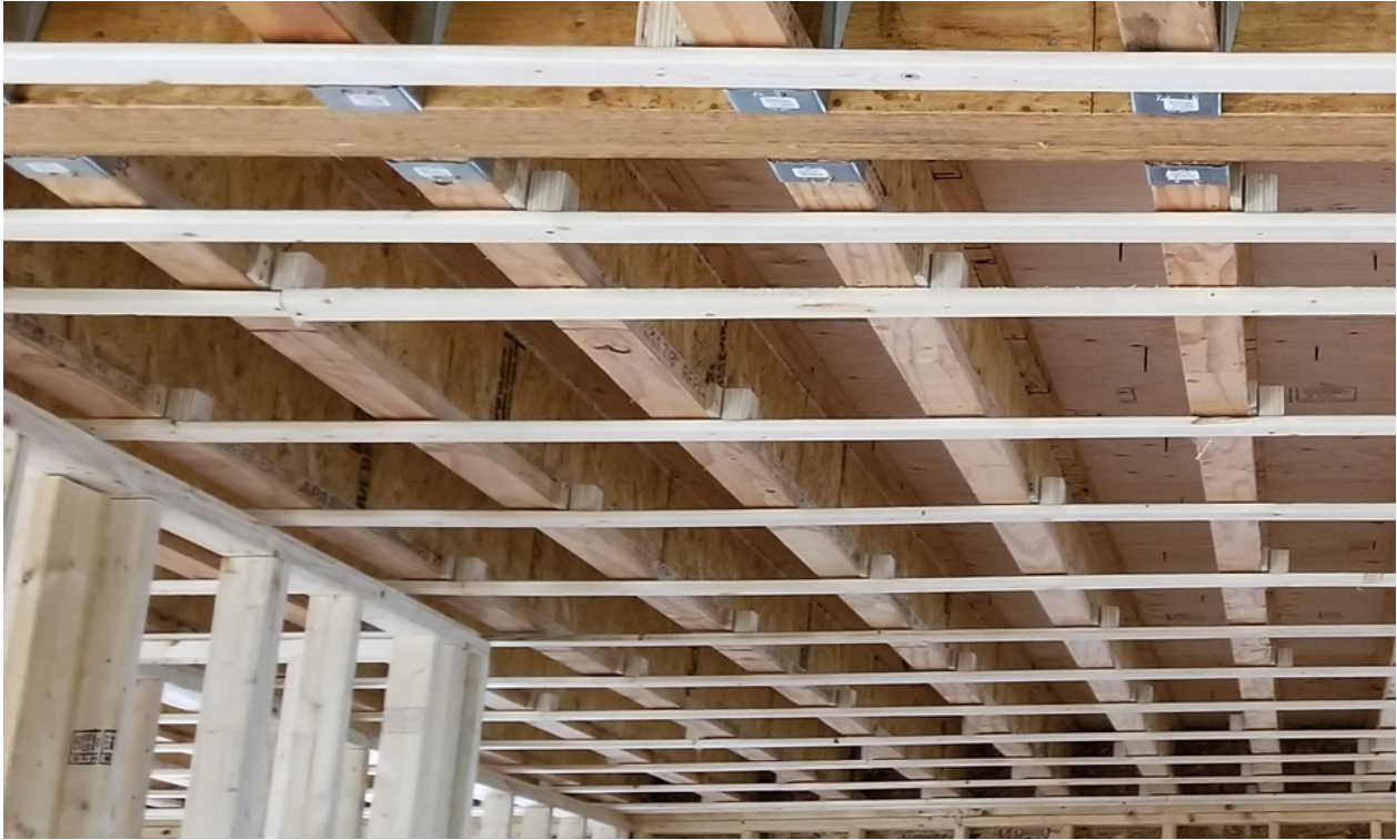
Wood furring installed on the ceiling.
