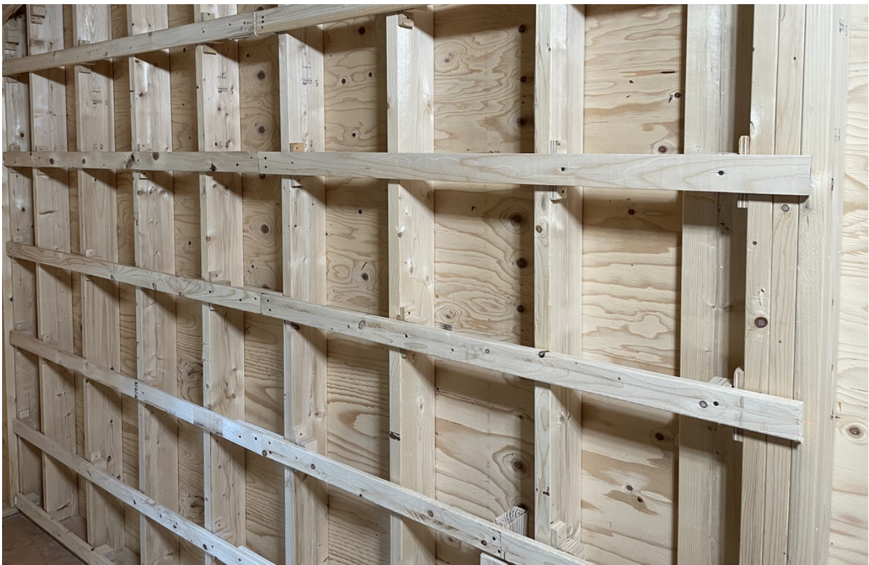
Wood furring installed on the wall.
