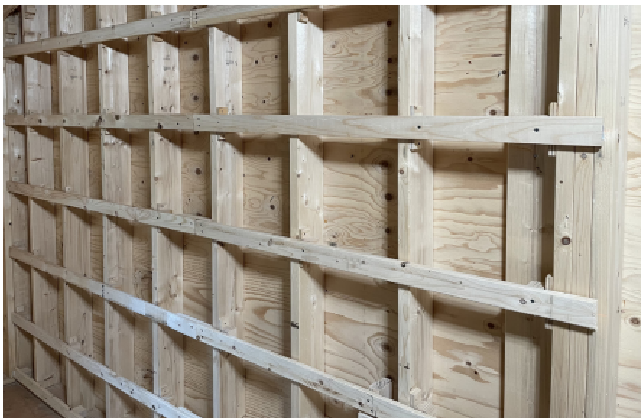
Wood furring installed on the wall.
