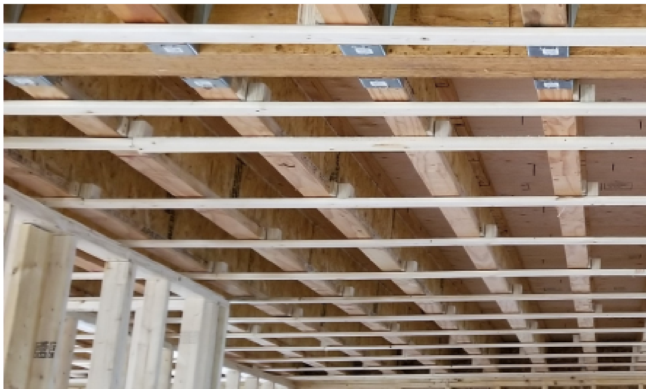
Wood furring installed on the ceiling.
