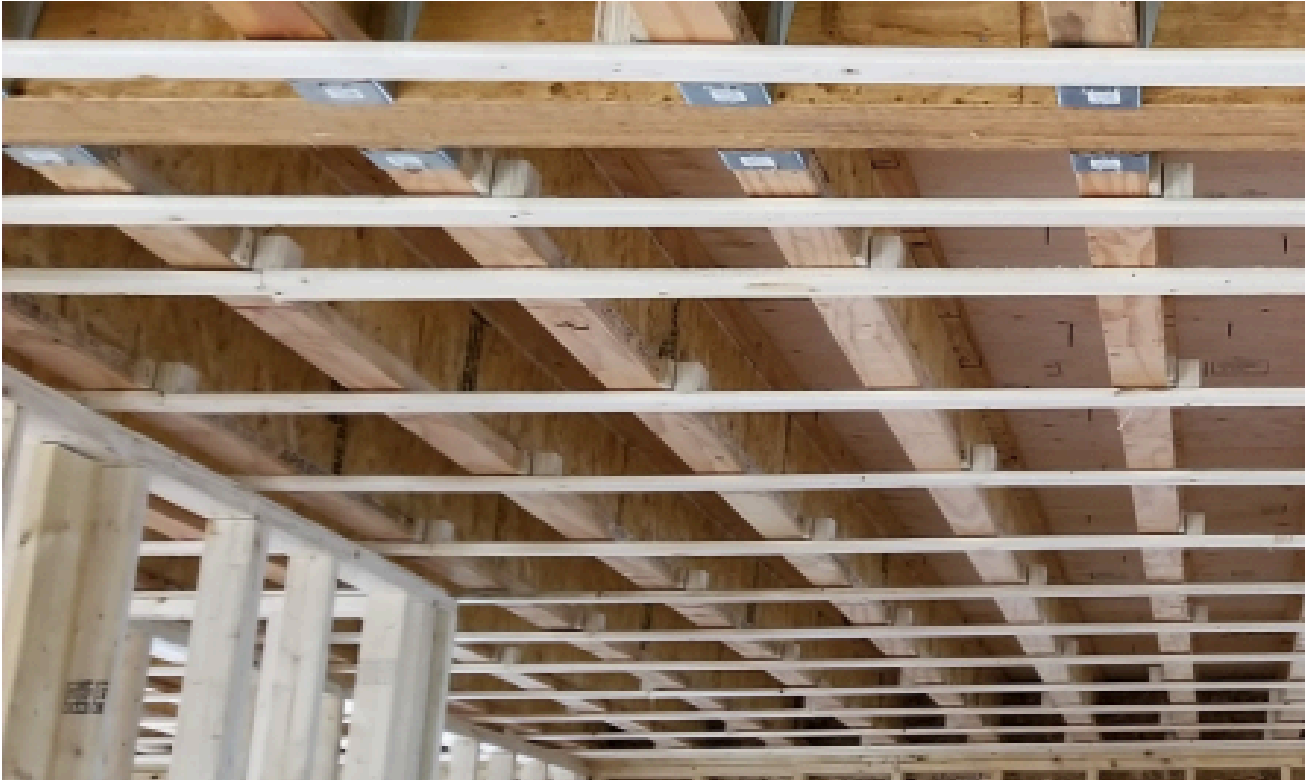
Wood furring installed on the ceiling.
