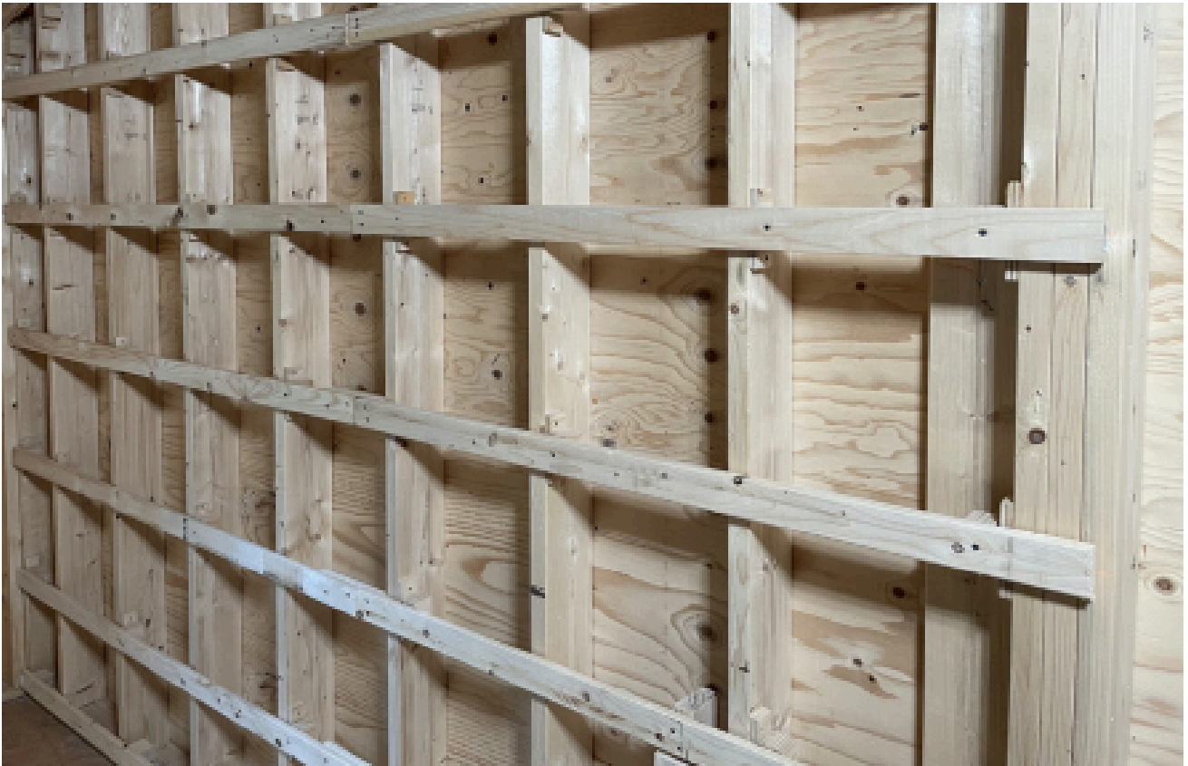
Wood furring installed on the wall.
